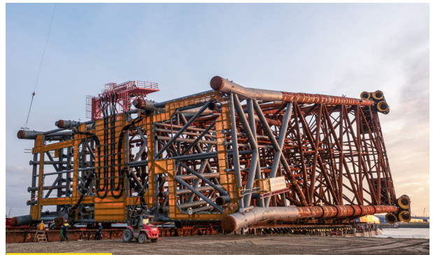
CONSTRUCTION OF THE PEREGRINO JACKET
