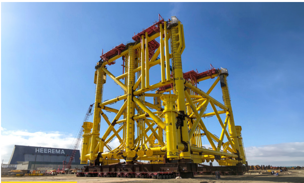
A SIX-LEGGED MAIN PILE JACKET
